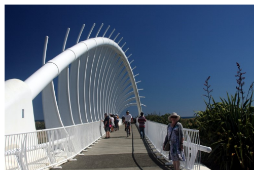
The Te Rewa Rewa Bridge
